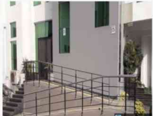
Wheel Chair and Ramp Access F Block
