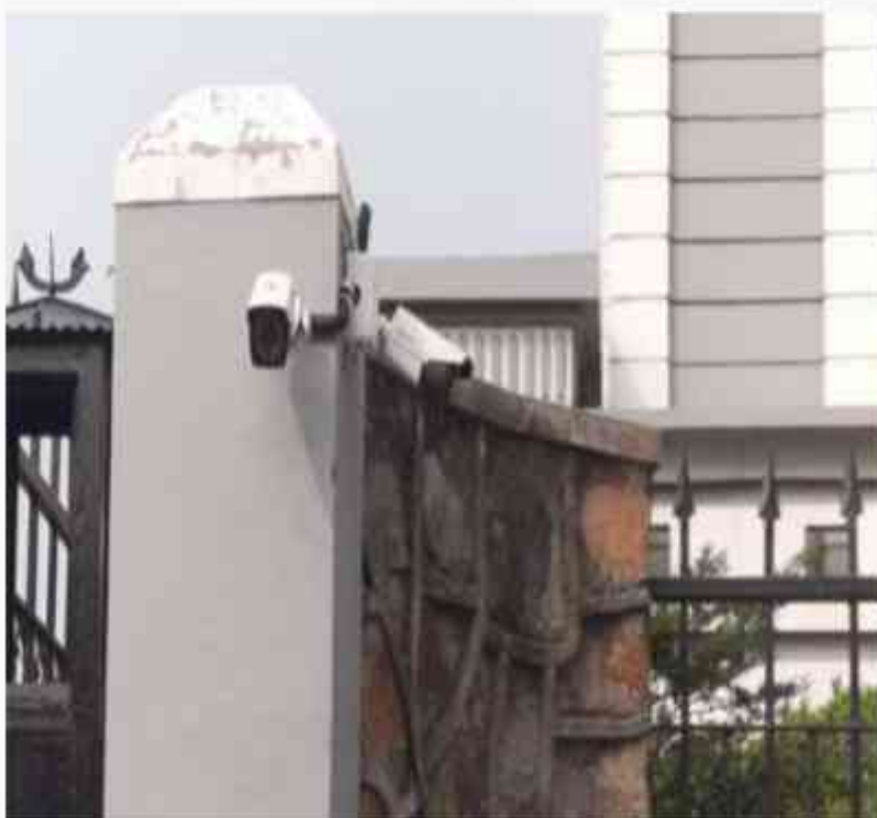
CCTV cameras outside buildings
